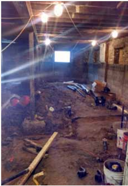
Basement had to be dug 12 inches deeper per building code. The digging was done manually. All plumbing has to be in place for inspection before cement is poured.
