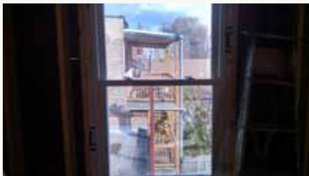
First new window installed on upper level.
