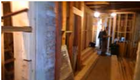
Structural beams and floor were laid before insulation and dry wall can go up.
